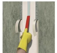
The adhesive top layer may be smoothed with a brush using a diluted detergent. Allow adhesive to start curing first.
