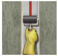
For fixing overhead or in difficult configurations, the tape may be temporarily held in place with Sika<sup>®</sup> Trocal Adhesive C-705. This adhesive, however may only be used in the tape centre but never on the areas to be bonded with Sikadur<sup>®</sup>-31 DW
